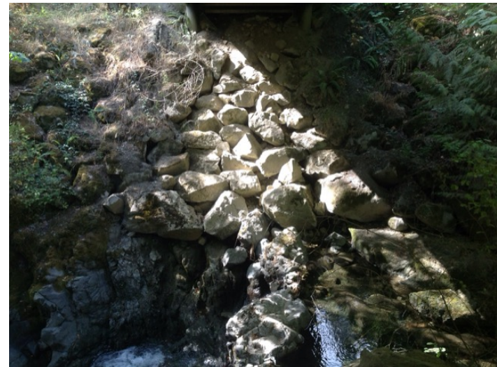
Right Bank Abutment when facing downstream
