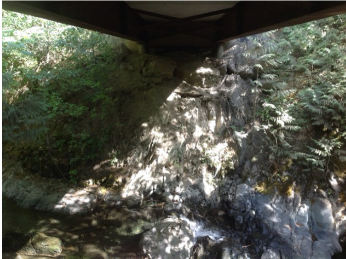
Left Bank Abutment when facing downstream
